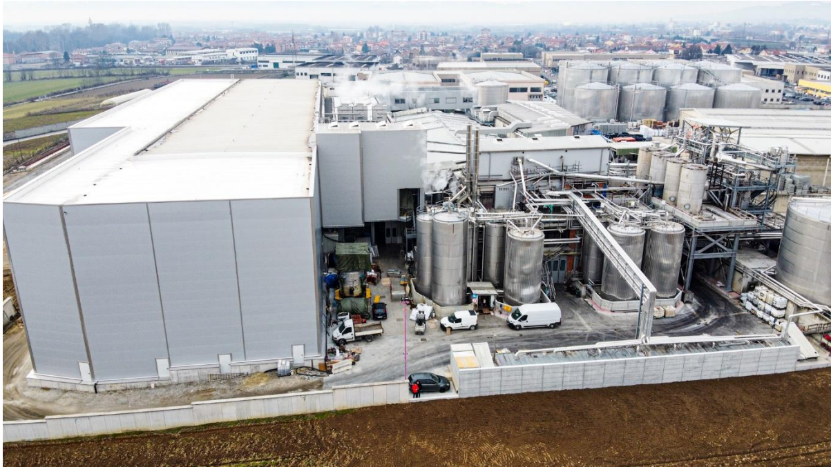
SER plant developments in progress
